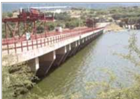
Figure 13: Part of the Mtera Dam
